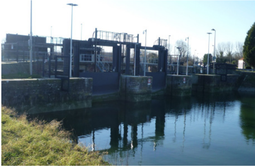
Wateringues territory, Gravelines structure: to evacuate water from the AA to the sea while avoiding marine intrusions Source : setec hydratec
